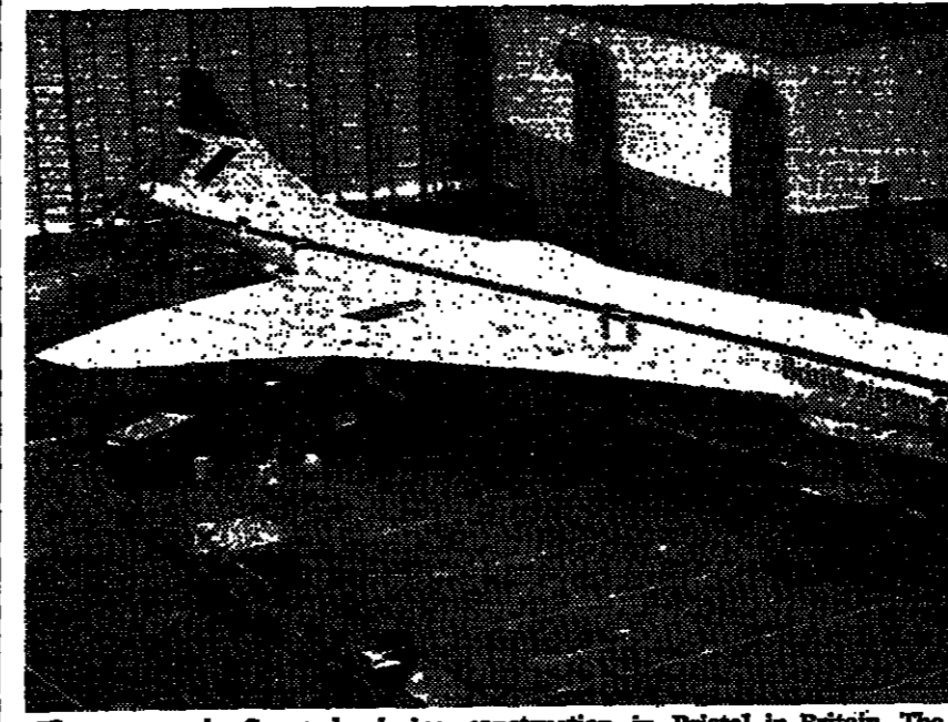
The supersonic Concorde during construction in Bristol in Britain. The British and French have agreed to put off building more Concorde after selling fewer than a dozen. They plan to build other types of aircraft.
